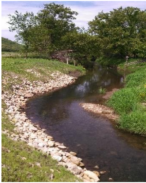
A rip rap project in the County
