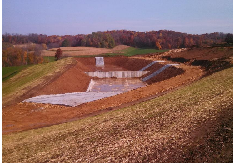
Manure Pit Construction
